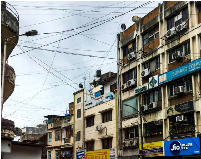
Tangled: Wiring of the buildings doesn't always seem to follow a plan. Here, many of the wires appear wrapped around other wires for support.
