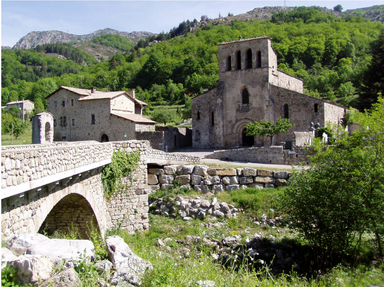
Photo 3: Picture of Our Lady of Provencheres Church in Montpezat.
